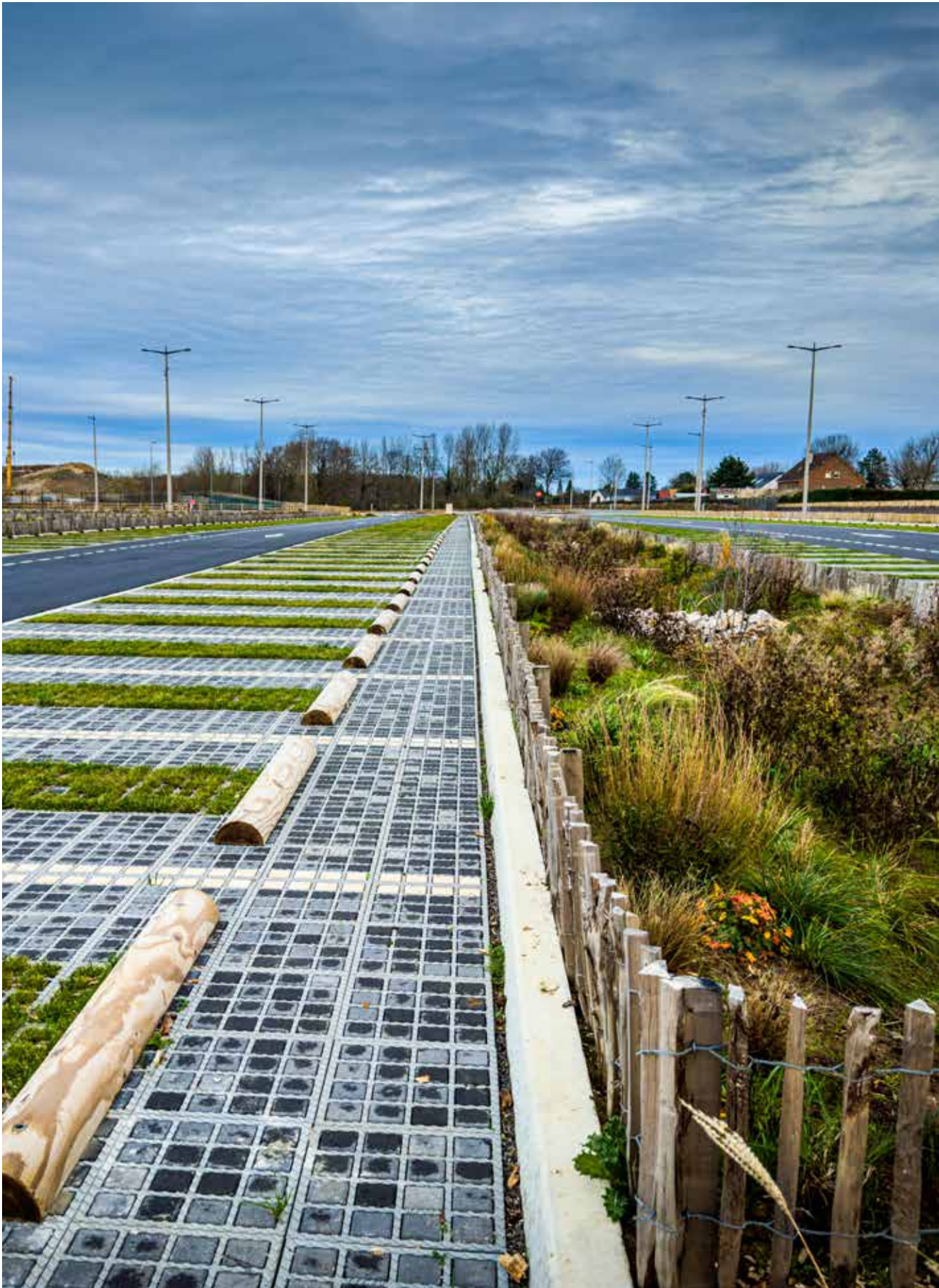
Chantier Penly parking central 2000 places - Penly (76)
